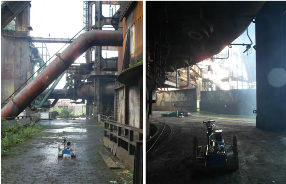
Figure 4: Impression of the “Phoenix West” former blast furnace, at which the T-JEx and T-Eval exercises took place.
